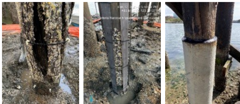
Figure 4. Progressive repair steps using the PileMedic® system.
