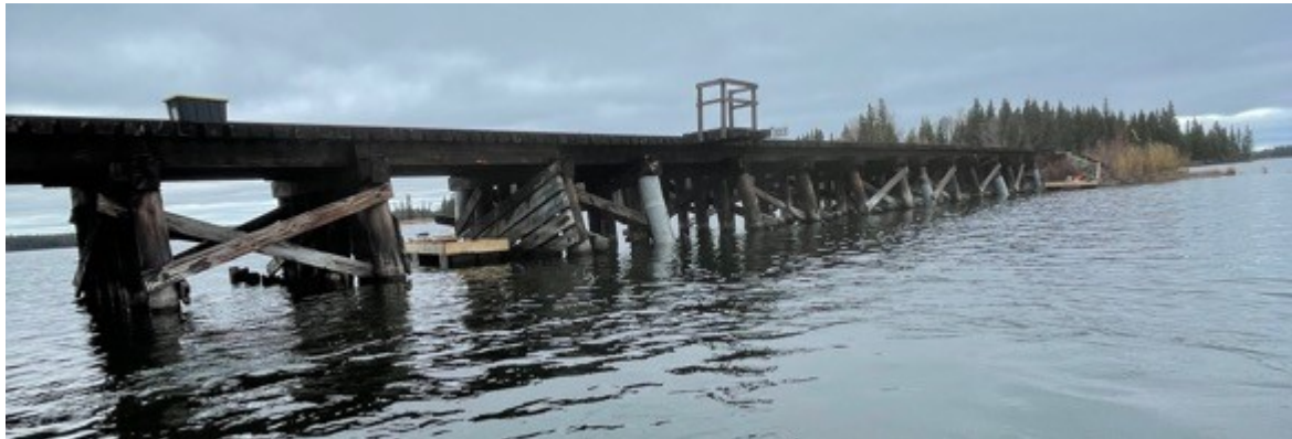
Figure 9. One of the rail bridge sites where dozens of piles were repaired.
