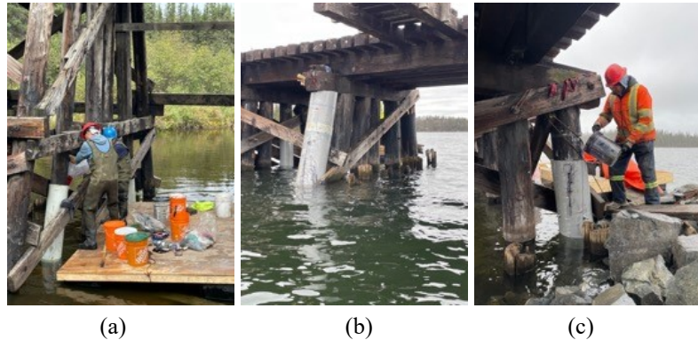
Figure 7. Installing the laminates to create a (a) partial or (b) full height repair of a pile; (c) placement of low viscosity resin in the annular space.
