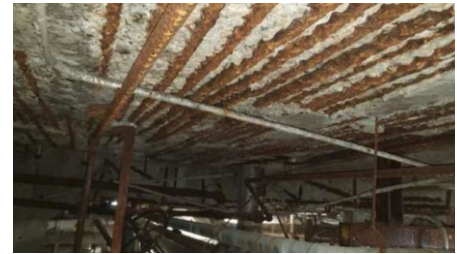
Fig. 9. Severely corroded slab in an industrial plant
