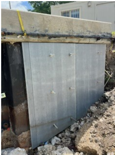
Fig. 6. Repair of corroded steel sheet piles in Weston, FL, June 2024
