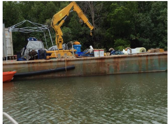
Figure 10 - Barge used as working platform
