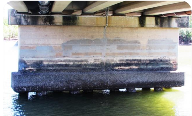
Figure 1 - View of typical pier
