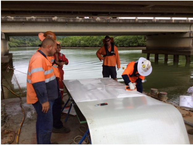
Figure 11 - Cutting of laminate to size and application of epoxy paste
