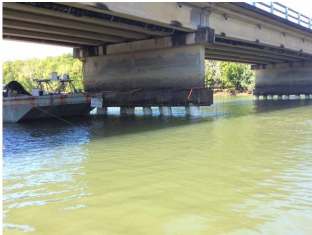
Figure 13 - Views of the completed project
