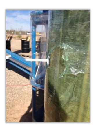
3. Inject our low viscosity resin to fill all the voids and cracks in the pole
