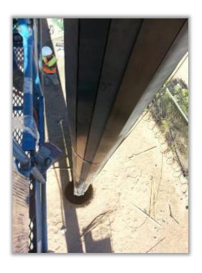
1. Provide longitudinal carbon strips along the height of the pole
