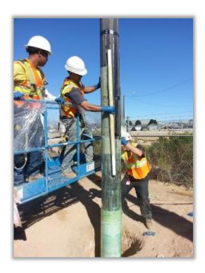
2. Wrap the pole with PileMedic<sup>TM</sup> laminates or QuakeWrap® FRP fabric
