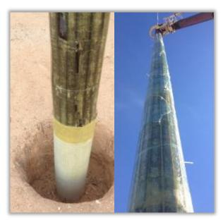
4. The repair covered the elevations from 2'-9" below ground to 25'-9" above ground. This procedure allows the pole to remain in service during the repair.
