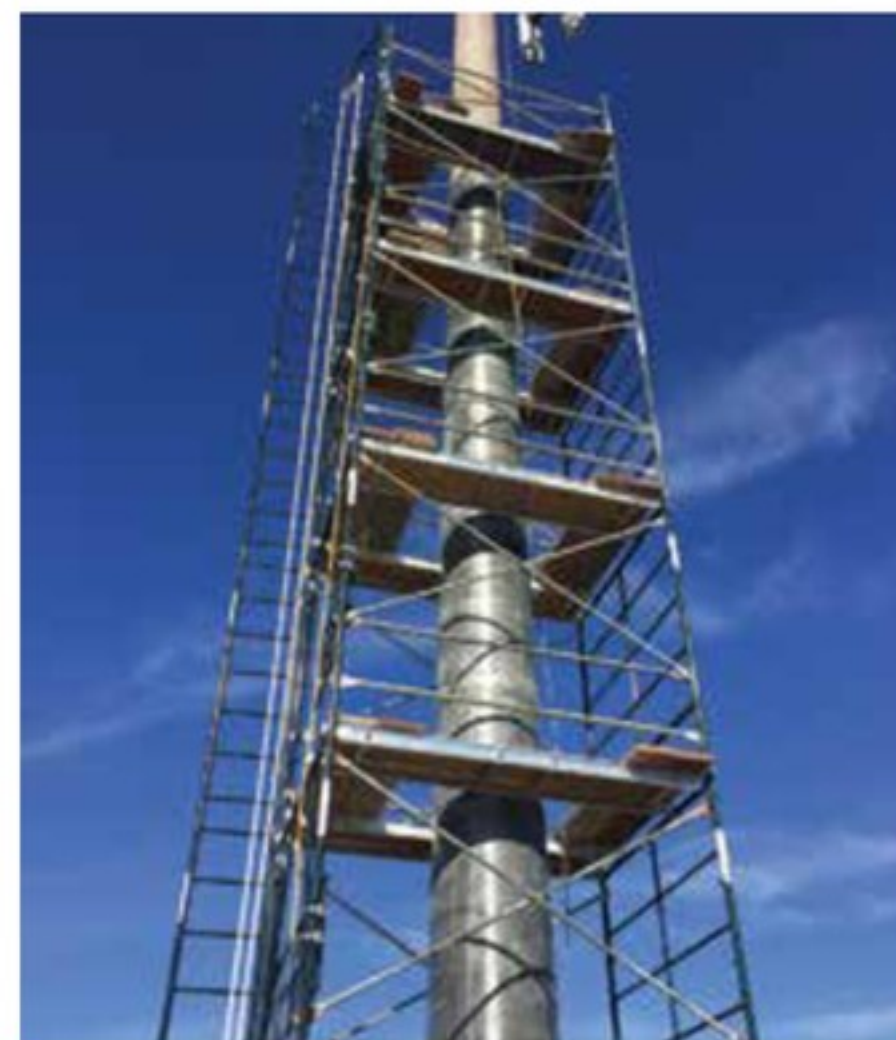
Figure 3. Carbon and glass FRP fabric applied to the lower 35 feet of the pole.
