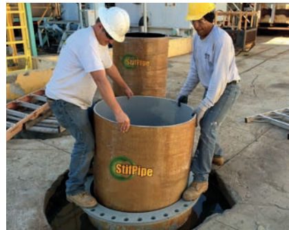
Insertion of StifPipe® into a Pressure Pipe Manhole at a Puerto Rico Power Plant
