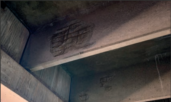
DAMAGED CONCRETE BEAM
