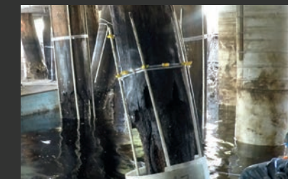
Spacers and FRP rebar attached to the pile
