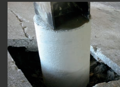
Section after strengthening with PileMedic®
