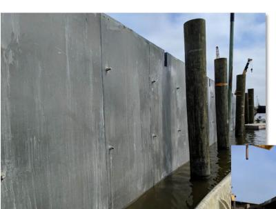
Installed SPiRe® FRP panels improve corroded steel sheet pile bulkhead.
