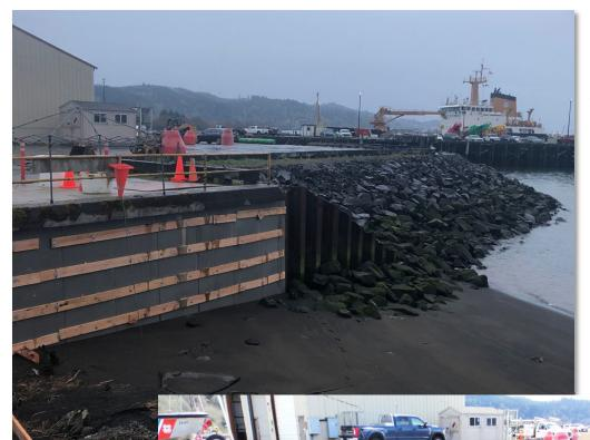
Repairs to steel sheet pile bulkhead using the SPiRe® by QuakeWrap system are at near completion, left, and completion, bottom.
