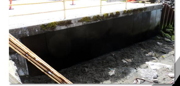
A black epoxy is applied upon completion of repair as requested by customer.
