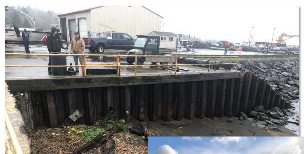
U.S. Coast Guard facility at Tongue Point, Astoria, OR, before and during repair of steel sheet pile bulkhead. Photos courtesy QuakeWrap Inc.
