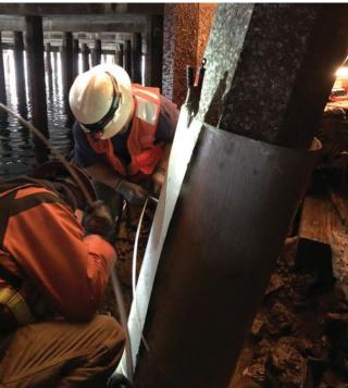
PILEMEDIC ENGINEERS DESIGNED AN EFFECTIVE REPAIR SYSTEM FOR THE PORT OF SEATTLE PILES THAT WOULD CALL FOR WRAPPING PILEMEDIC LAMINATE JACKETS COMPLETELY AROUND THE PILES.
