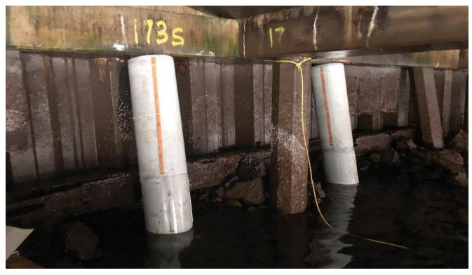
he current repair work — scheduled for completion at the end of 2017 — involves the retrofit of 40 prestressed driven piles of varying length located under T-18. No shutdown of service was needed during repair, with more than half of the piles 30 feet or longer, and in varying degrees of water submersion.
