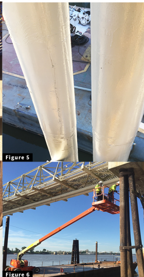
Figure 1, Figure 2, Figure 3, Figure 4, Figure 5: Use of spacer between PileMedic jacket and voided timber piles, Figure 6: Access to the timber piles from the barge,
