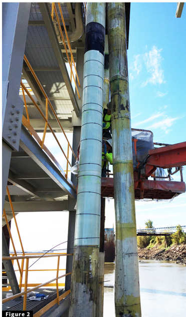
Figure 1, Figure 2, Figure 3, Figure 4, Figure 5: Use of spacer between PileMedic jacket and voided timber piles, Figure 6: Access to the timber piles from the barge,
