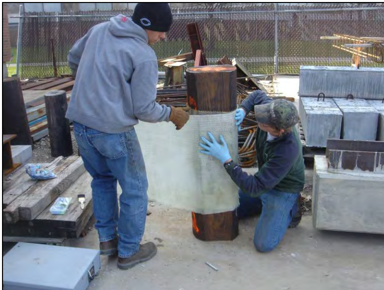
Figure 13.9. Wrapping the FRP sheet around the timber pile
