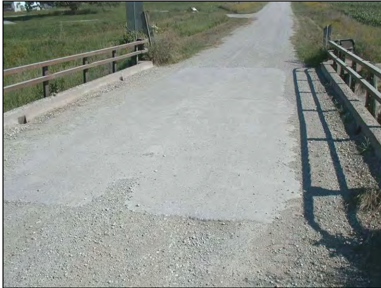
Figure 9.1. Bridge No. 237350 – Looking north (October 25 2005)
