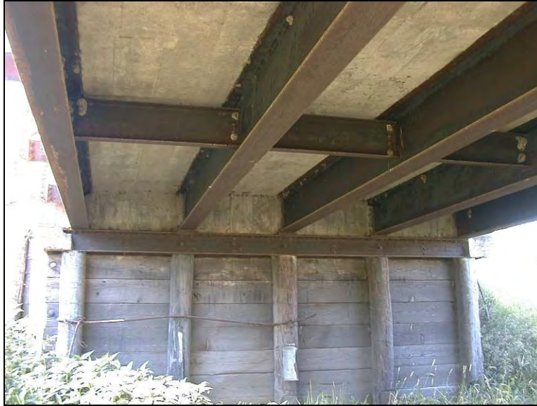
Figure 9.6. South abutment (Bridge No. 237350 Mahaska County – October 25 2005)
