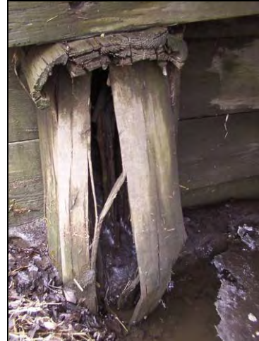
(b) Complete deterioration of pile section (Bridge No. 27-42-00 Buchanan County – February 16 2005)
