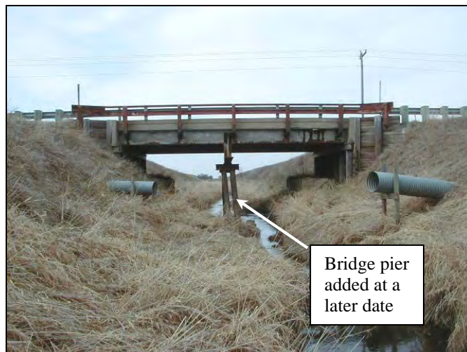
Figure 12.2. Center pier added in the 1970s (Bridge No. 029070 Humboldt County – April 4 2006)
