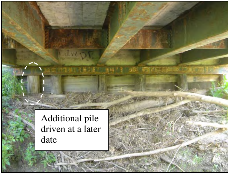
Figure 8.3. North abutment (Bridge No. 243470 Marshall County – July 22 2005)
