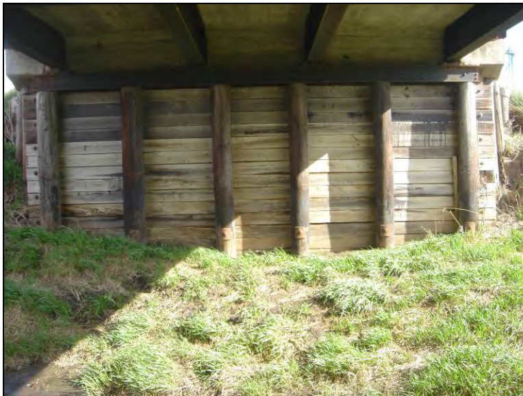
Figure 10.5. North abutment (Bridge No. 094680 Carroll County – April 15 2006)
