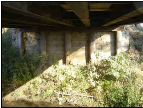
(a) Overview of the north abutment before replacement
