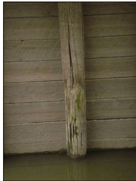
(b) Pile no. 3
