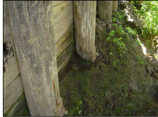
(b) Pile no. 4
