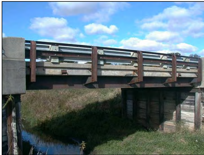
Figure 10.1. Side view of the bridge looking northwest (Bridge No. 094680 Carroll County – May 16 2006)
