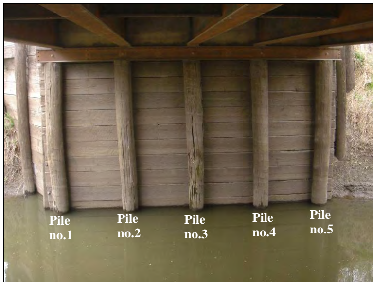
Figure 11.3. Northwest abutment (Bridge No. 237380 Mahaska County – April 16 2006)
