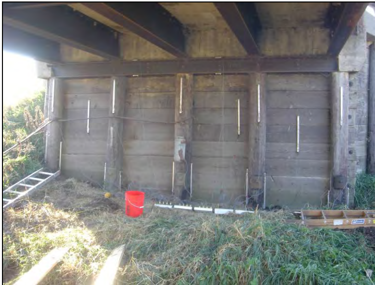
(b) South abutment
