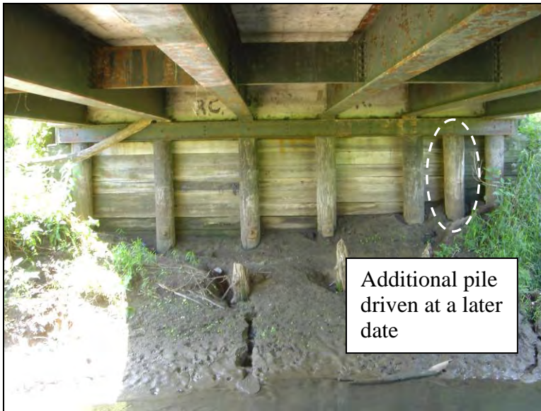
Figure 8.4. South abutment (Bridge No. 243470 Marshall County – July 22 2005)
