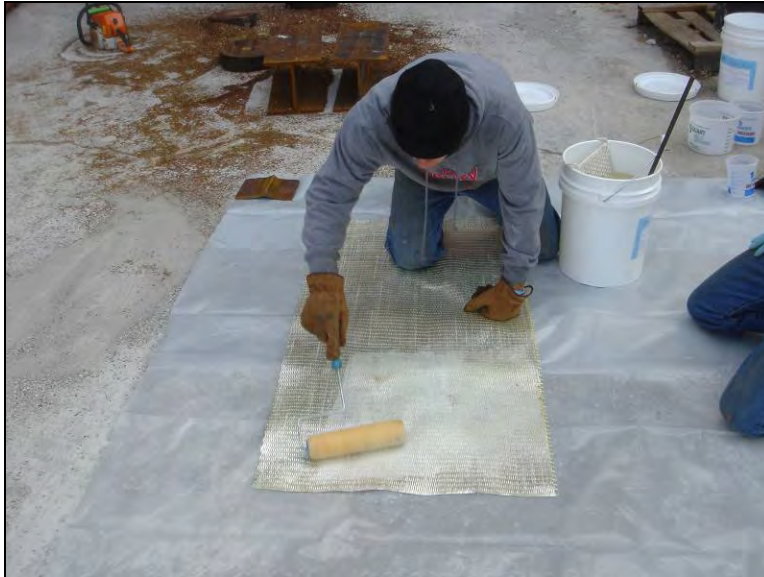
Figure 13.8. Applying the bonding epoxy using a paint roller
