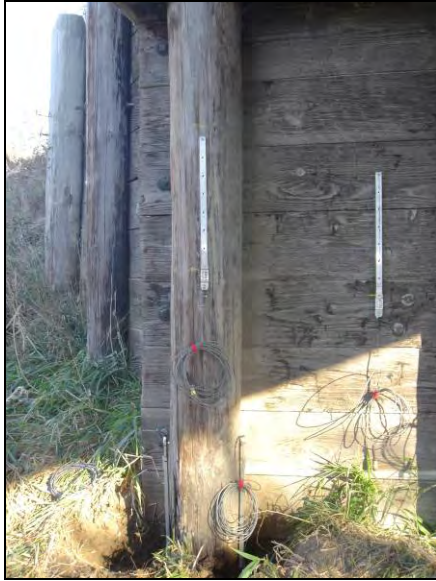
(a) Pile no. 1 at the north abutment
