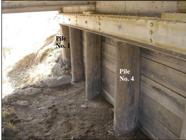
Figure 12.10. West abutment (Bridge No. 029070 Humboldt County – April 4 2006)
