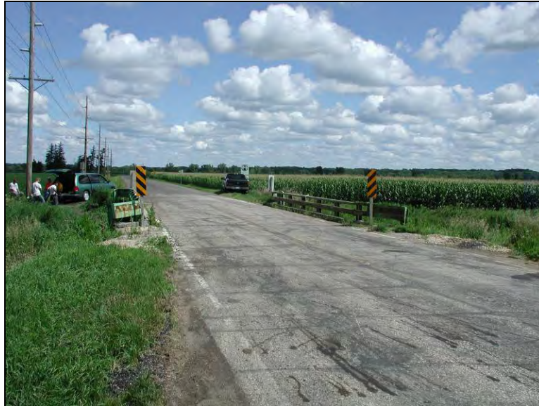
Figure 8.1. North view of Marshall County Bridge No. 243470 (July 22 2005)
