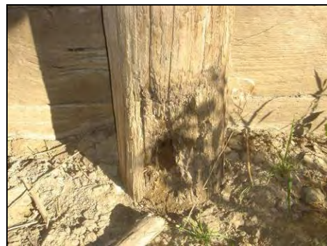
(d) hollow pile section near the ground level
