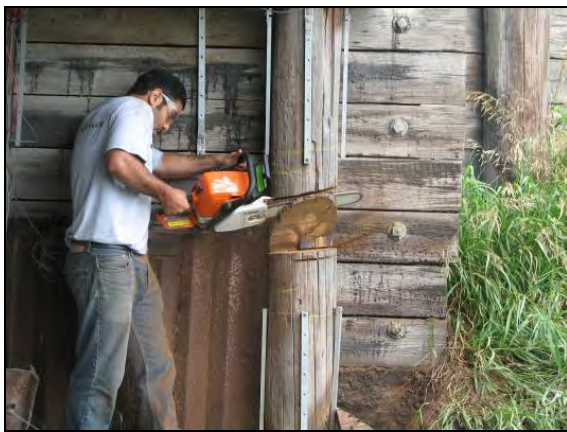
(a) Removing pile no. 7
