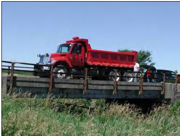
Figure 6.1. Tandem axle truck using to carry out static load tests
