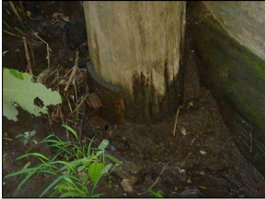
(a) Pile no. 1
