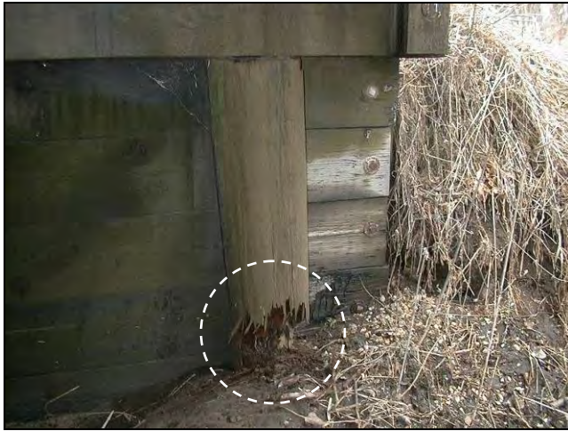
(a) Reduction of pile cross section (Bridge No. 13-42-06 Buchanan County – February 16 2005)
