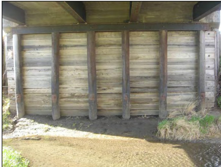
Figure 10.7. South abutment (Bridge No. 094680 Carroll County – April 15 2006)
