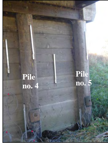
(b) Pile nos. 4 and 5 at the south abutment
