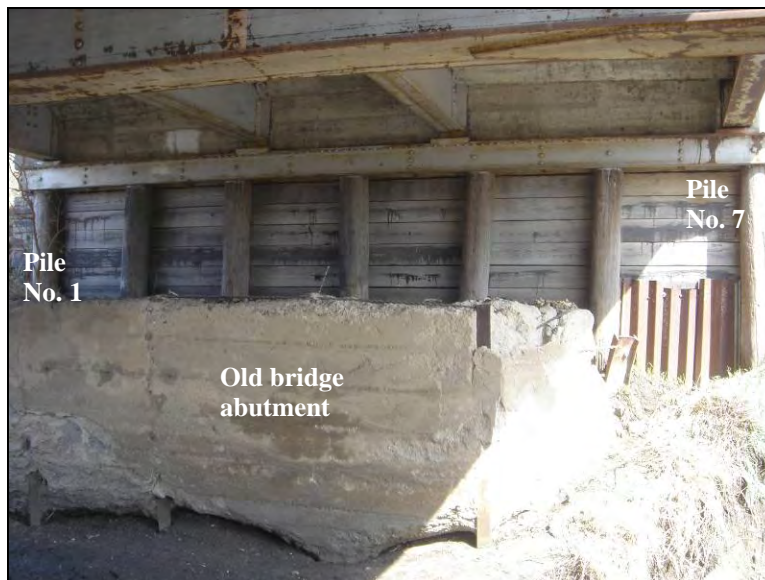
Figure 12.7. East abutment (Bridge No. 029070 Humboldt County – April 4 2006)
