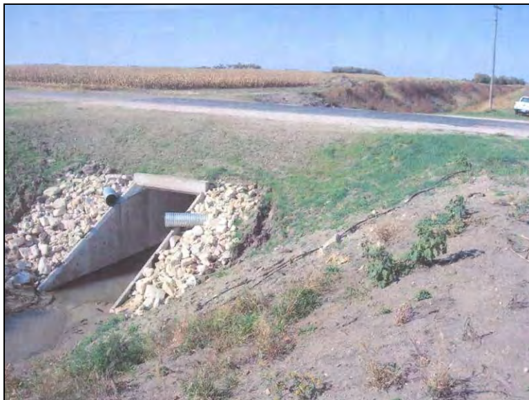
Figure 12.13. New box culvert – view looking north (Bridge No. 029070 Humboldt County – October 5 2006)
