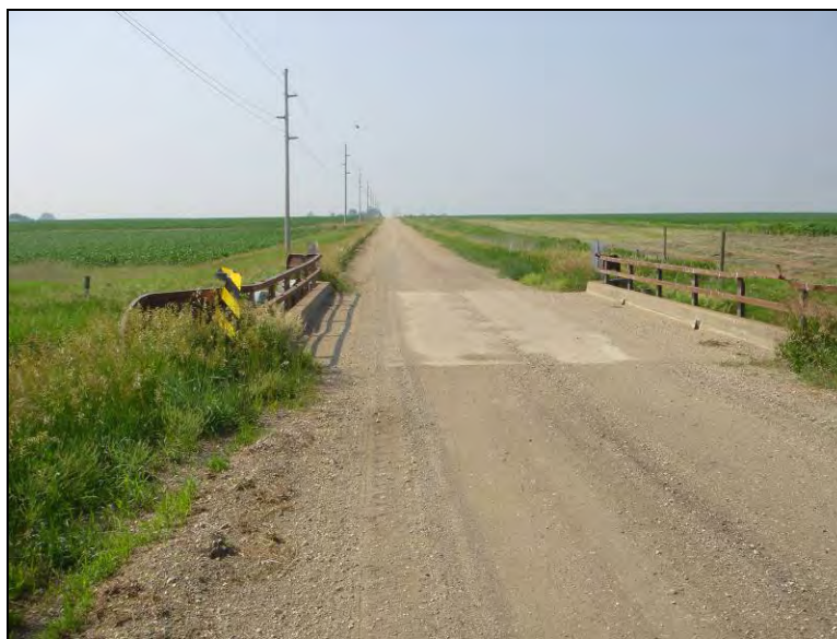
Figure 7.1. Bridge No. 7710 Boone County – looking south (June 24 2005)
