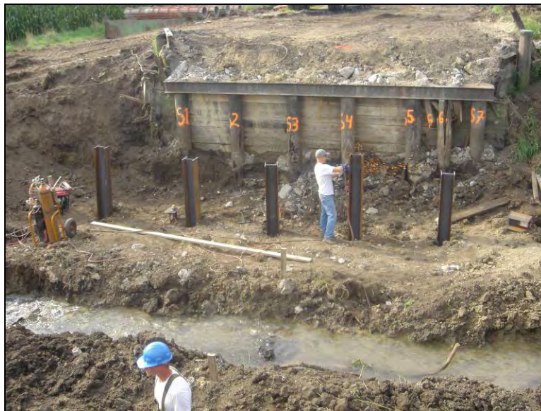
Figure 8.9. Construction of the new bridge foundation (Bridge No. 243470 Marshall County – August 19 2005)
