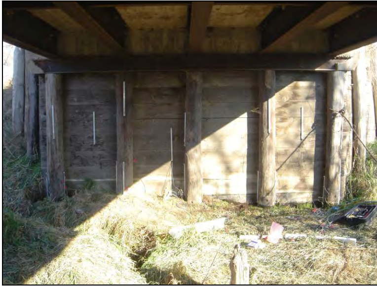
(a) North abutment
