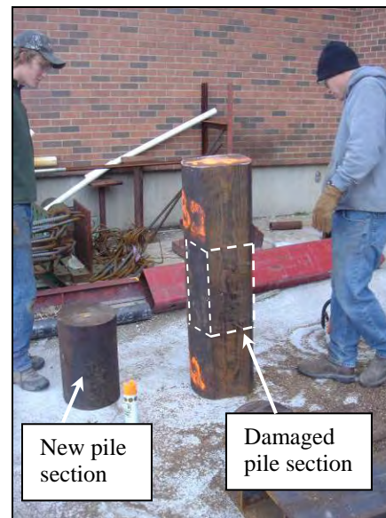
(b) Replacing old timber section with new one
