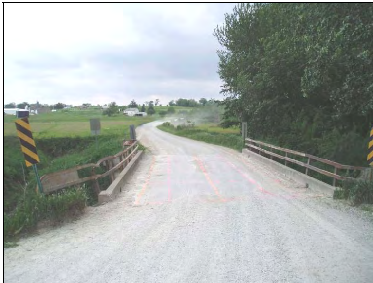
Figure 11.1. Bridge No. 237380 – Mahaska County (April 16 2006)
