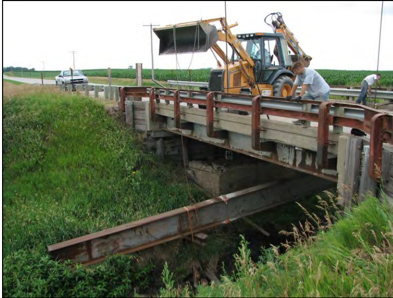
Figure 12.5. Lowering the steel girder (Bridge No. 029070 Humboldt County – July 10 2006)
