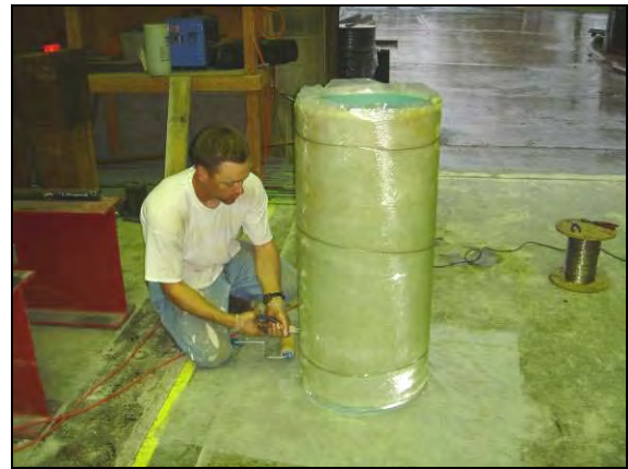
(b) FRP sheets wrapped around the pipe
