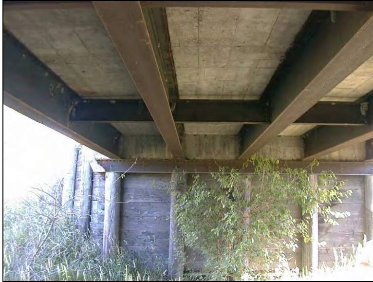
Figure 9.2. North abutment (Bridge No. 237350 Mahaska County – October 25 2005)
