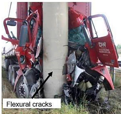
Fig. 1. Real-world bending deformation due to an impact event [32]
