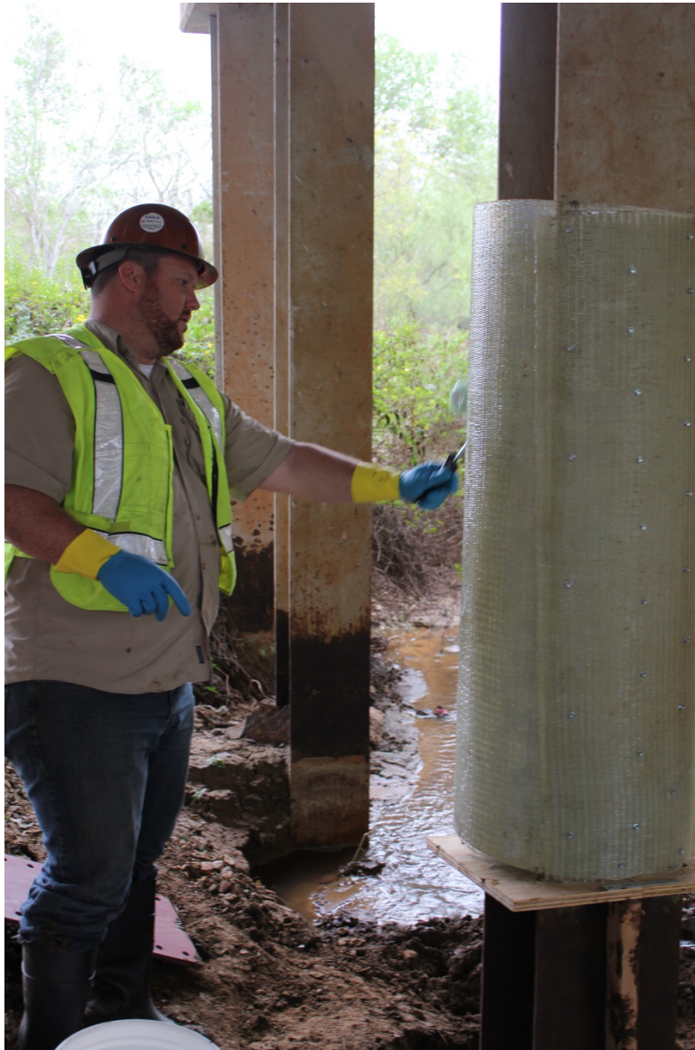
Figure 12.6: Coating the GFRP jacket with epoxy
