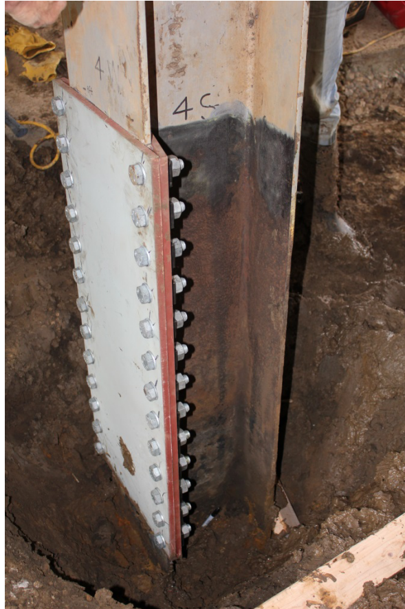
Figure 12.12: Steel based repair system
