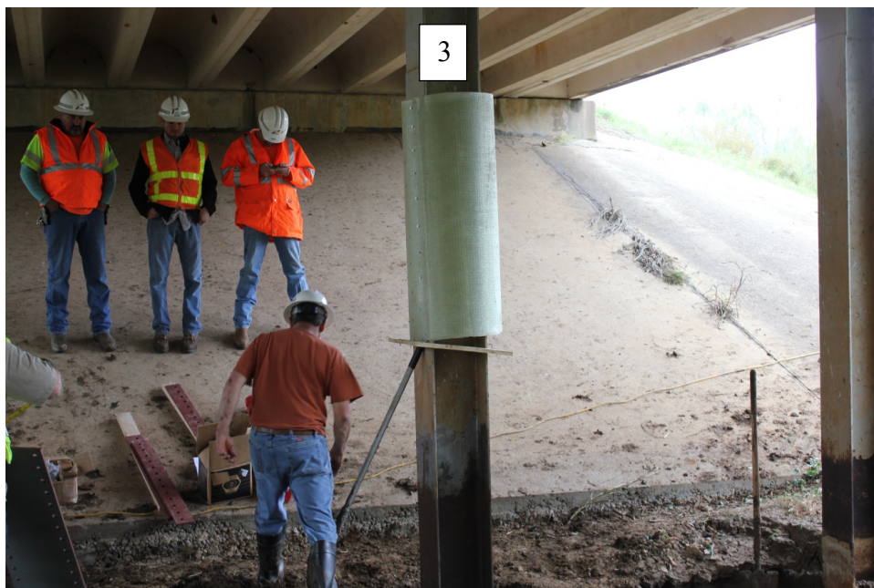
(b) Positioning of GFRP jacket on pile 3
