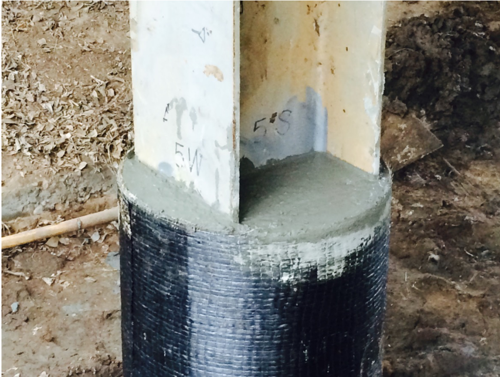
Figure 12.8: Completed installation of grouted FRP-jacket
