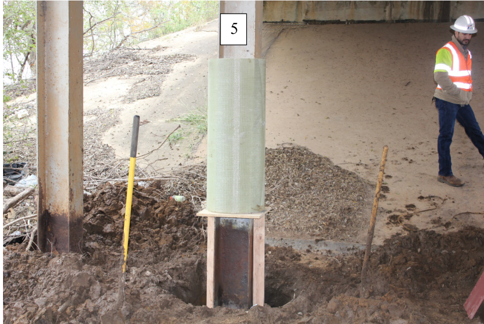
(a) Positioning of GFRP jacket on pile 5
