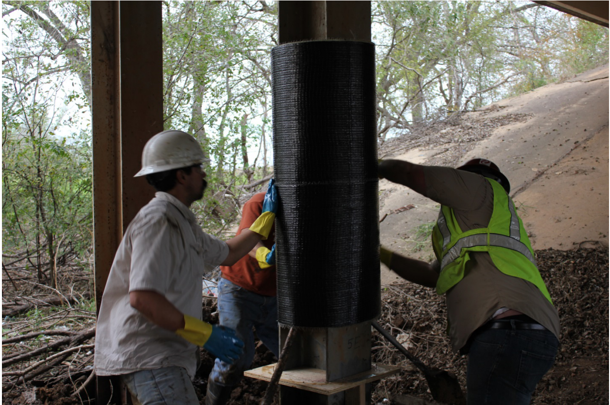
Figure 12.7: Installation of the CFRP overwrap
