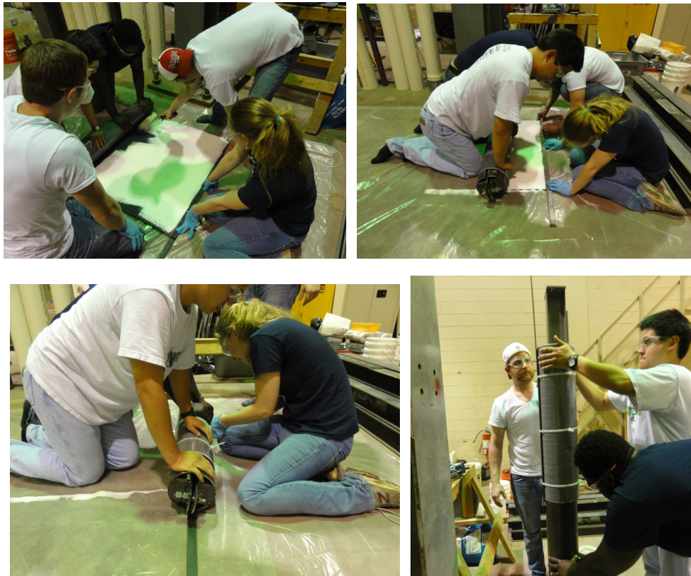
Figure 10.10: Fabrication of FRP jackets for Repair System 1
