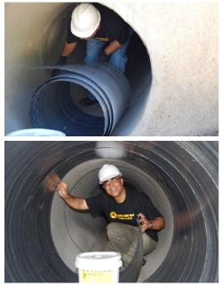
Figure 3: Coiled PipeMedic™ laminate being taken into a pipe and bonded to the pipe surface.
