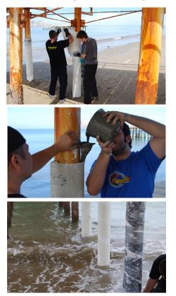
Figure 6: Construction of a continuous PileMedic™ jacket around an existing steel pipe with super laminate; filling the annular space with grout, and view of retrofitted piles.
