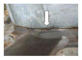
Close-up - Crack Near Weld that Joins the Pole to its Base Plate
