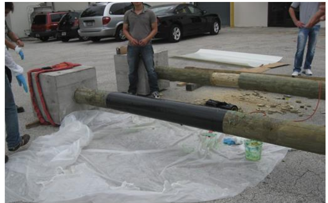
Figure 4.5: Holding GFRP sheet around the pile by Saran TM plastic wrap
