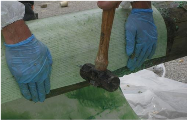
Figure 4.4: Wrapping GFRP sheet around the pile
