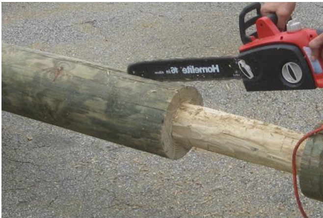
Figure 4.3: Preparing pile for GFRP sheet
