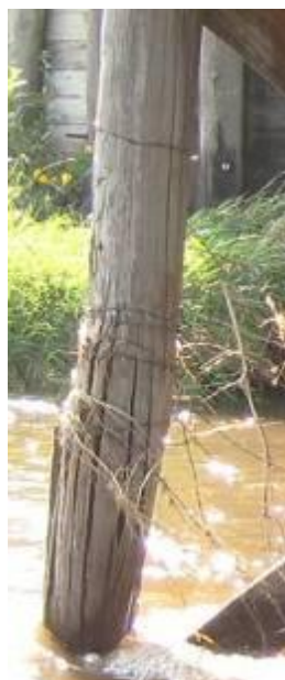
(b) Debris Damage
