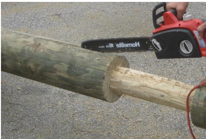
Figure 4.3: Preparing pile for GFRP sheet
