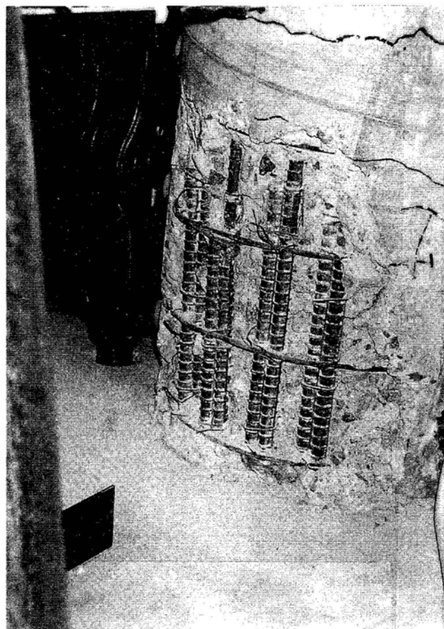
Fig. 22—Bond failure of Column C-1
