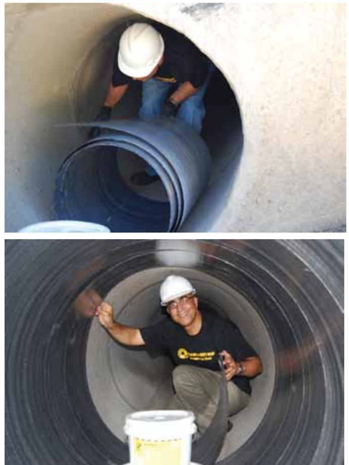
**Fig. 2: Super laminate being taken into the pipe and installed; one size fits all pipe diameters**
