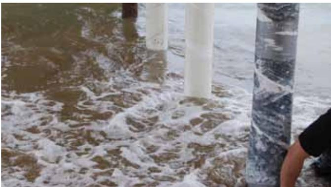
**Fig. 5: Retrofit of underwater piles, from top to bottom: construction of a seamless jacket with super laminates; filling the annular space; and completed pile jacket**
