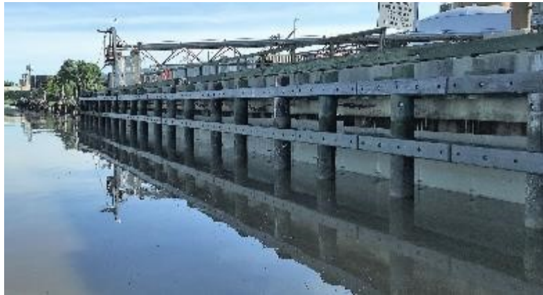
Fig. 4. Completed installation prior to placement of grout
