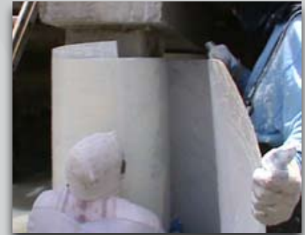
Wrap PileMedic™ around deteriorated pile to create a double-layer cylindrical jacket
