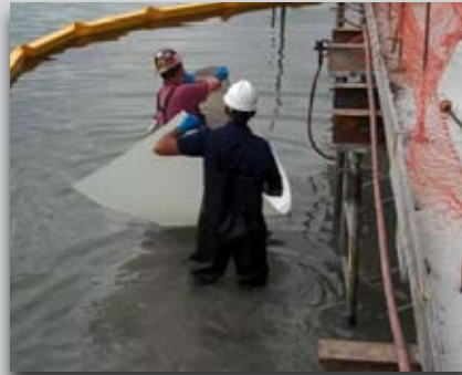
Transport the PileMedic™ sheet into water
