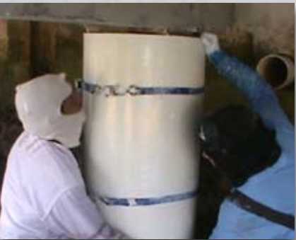
Temporarily support the jacket by wrapping a couple of ratchet straps around it
