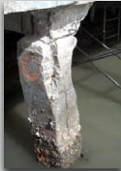
Deteriorated Pile
