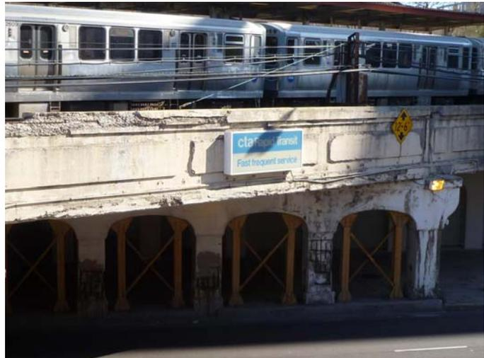
*Fig. 1. Corrosion-damaged concrete piles in Chicago being assisted with steel trusses*
