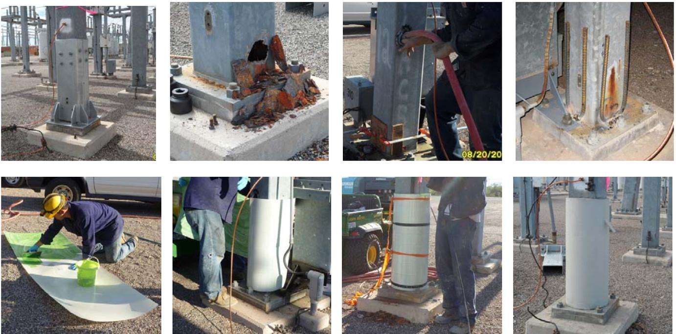
*Fig. 3. Repair of steel poles at TEP substations: original repair concept; corroded pole; filling the pole with grout; reinforcing steel welded to base plate; applying epoxy to the laminate, wrapping it around the pole and holding it with straps while grout is placed; finished and painted jacket*
