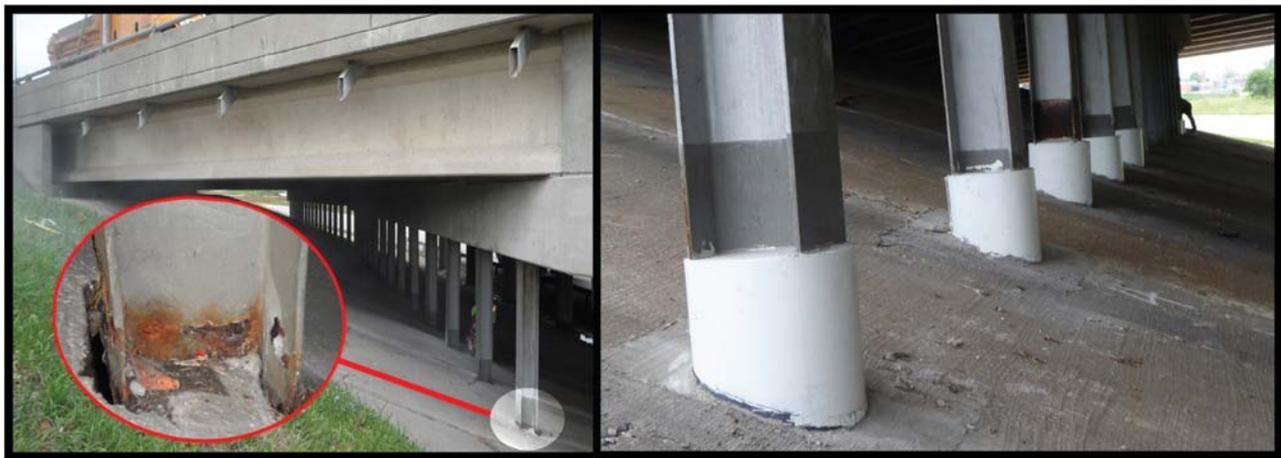
*Fig. 4. The I-70/I-270 interchange in St. Louis, MO where 49 corroded bridge piling were recently repaired with PileMedic™ jackets.*
