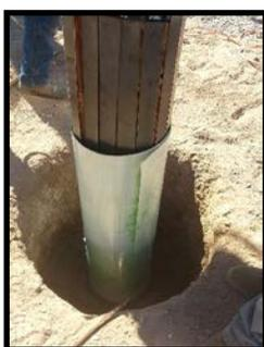
*Broken pole being repaired with Carbon FRP and PileMedic™*
