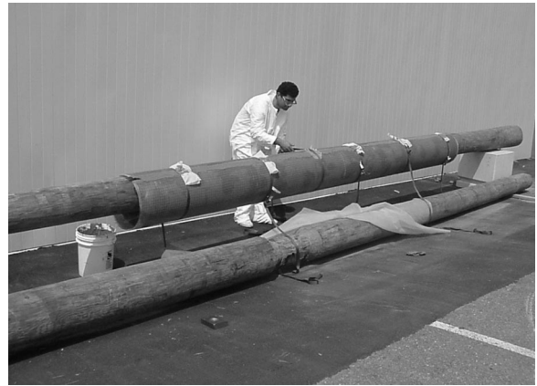
Fig. 11. Application of fiber-reinforced polymer composite shells to predamaged wood pile
