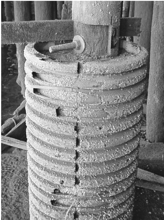
Fig. 4. Repair method using HDPE pipe encasing and splicing with steel bolts
