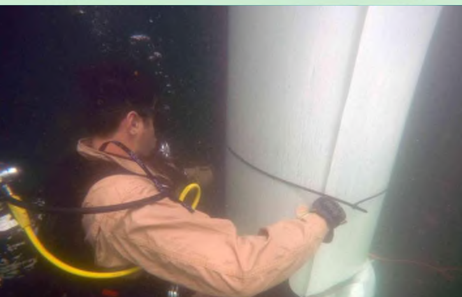
Diver Secures Laminate with Zip Ties
