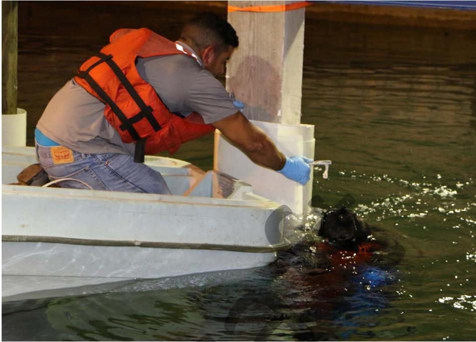
Figure 10. Divers place wrap on pile
