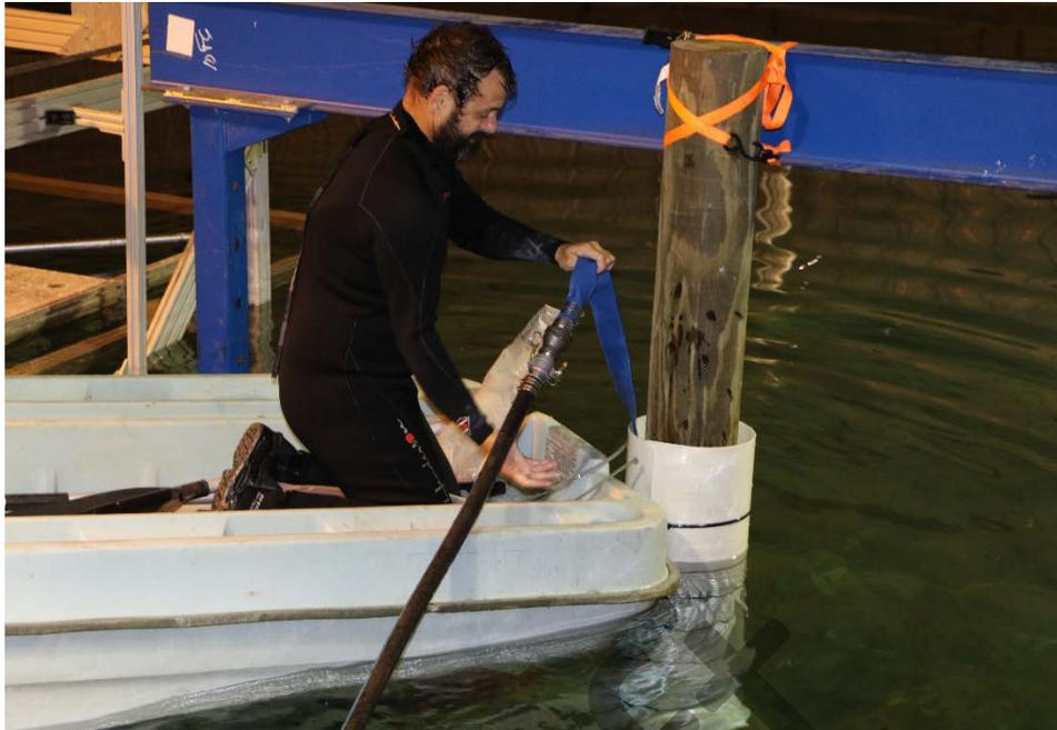
Figure 12. Placing grout in prepared jacket
