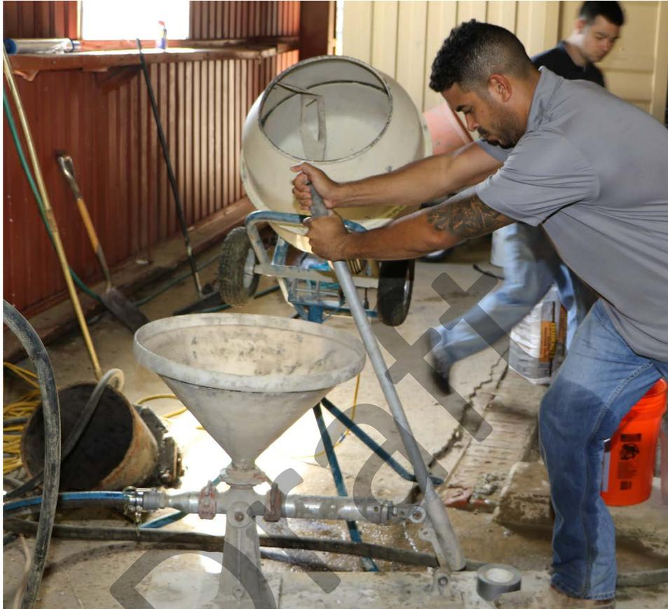
Figure 11. Hand pump used for grouting during the TD
