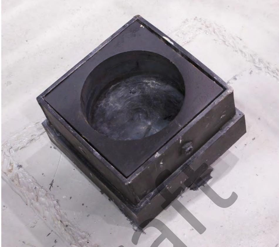
Figure 27. Timber column end cap
