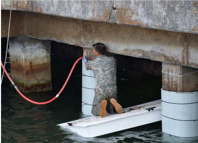
Figure 86. Grout placement
