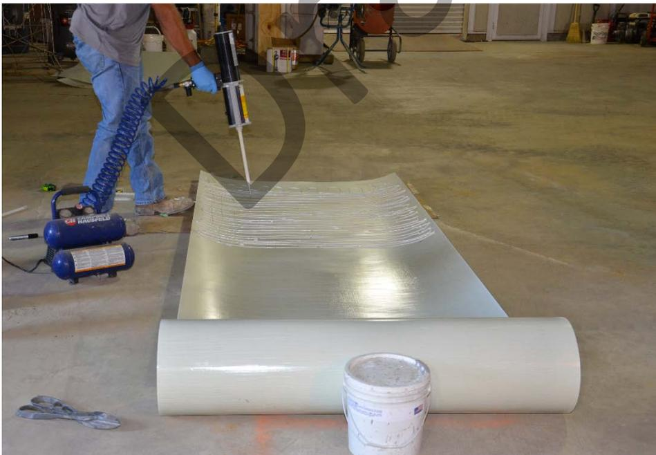
Figure 6. Applying epoxy to wrap using pneumatic dispenser gun
