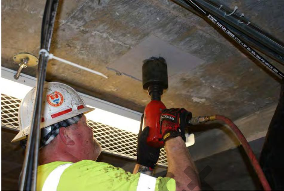
Figure 16. Tightening of nuts and securing the support to the strong floor
