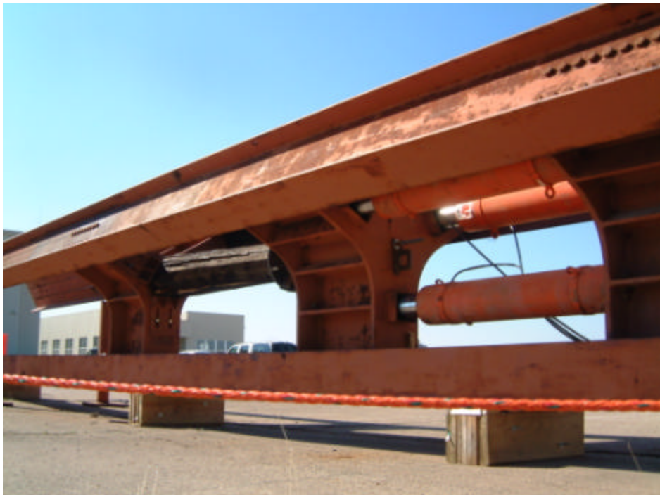
Fig. 1.3 Steel frame used in previous destructive tests
