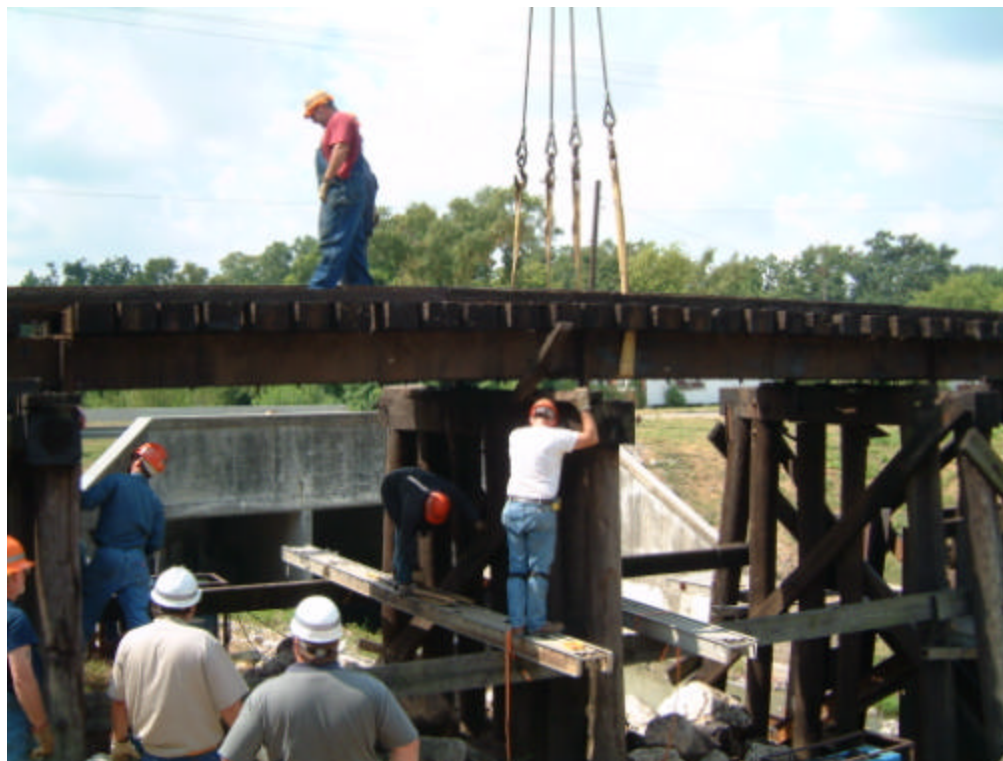
Fig. 2.7 Photograph of load cell installation with crane
