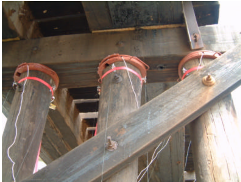
Fig. 2.6 Photograph of eye bolt anchor underneath bent cap
