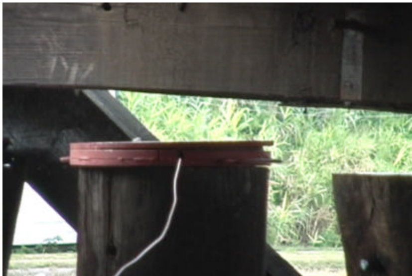
Fig. 2.2 Photograph of load cells in steel bearing plates
