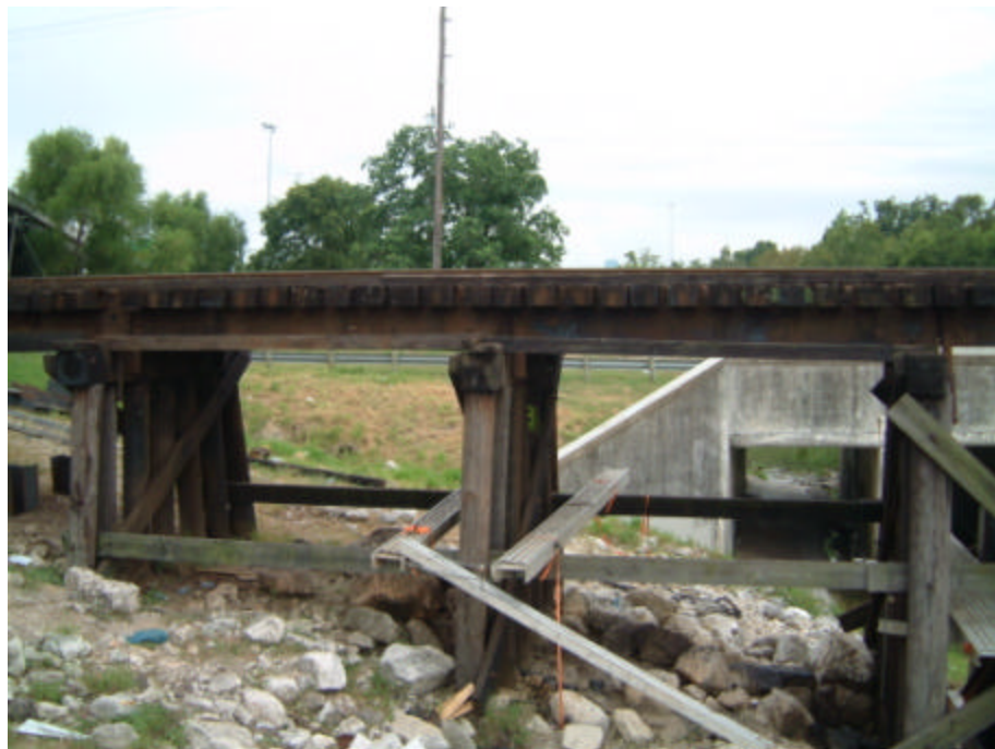
Fig 1.2 Lateral view of piles
