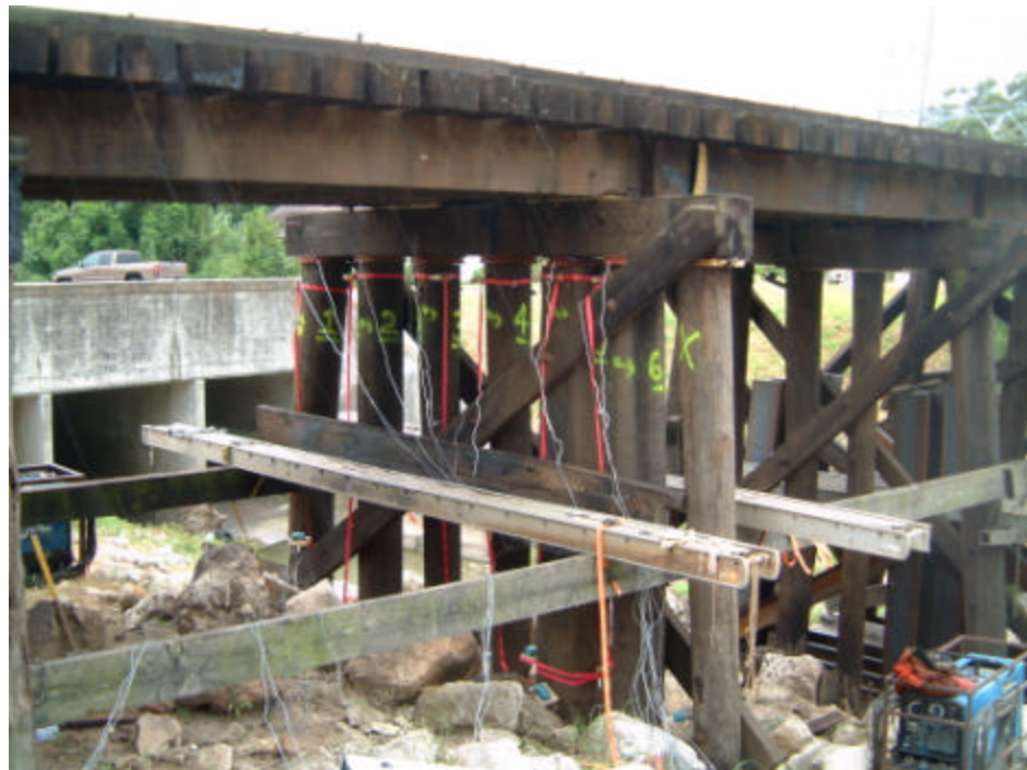
Fig. 2.4 Photograph of piles with identification labels
