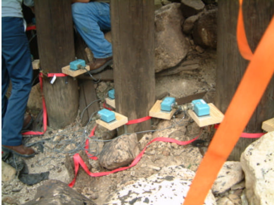
Fig. 2.5 Photograph of string pots installed on pile near the ground surface
