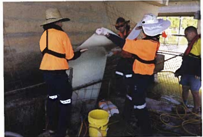
Fig. 4: Coated laminate being passed to the diving crew for installation
