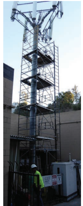
Fig. 7: Retrofitted pole prior to the application of paint and removal of the scaffolding
