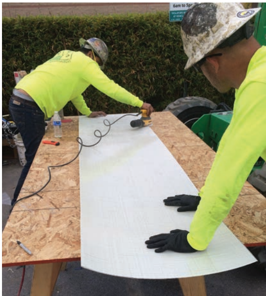
Fig. 5: FRP laminates used to create a shell around the pole
