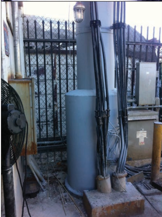
Fig. 6: Reinforcement detail near the base showing the anchored steel, FRP laminate shell, and the finished installation
